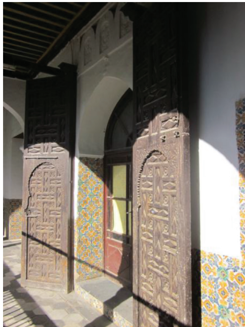
Figure 7: A view of a door of a main room.
