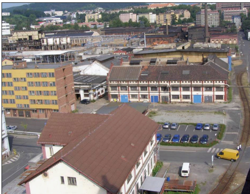
Figure 3: View of the former company Spolchemie.
