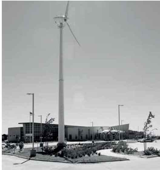
Figure 4: Post-tornado Hospital (photo by Joah Bussert).
