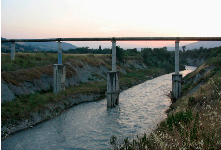
Figure 5: In 2004 the pile foundation was uncovered by 8 m.
