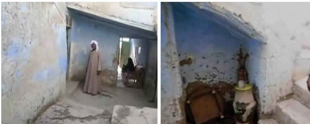
Figure 7: Inner courtyard in a house in Gournia, a social hub and a source for natural lighting and ventilation. Source: www.youtube.com .
