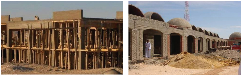
Figure 21: The local building materials have been replaced by conventional building materials from RC and Red Brick and were imported to the region and replaced [10].
