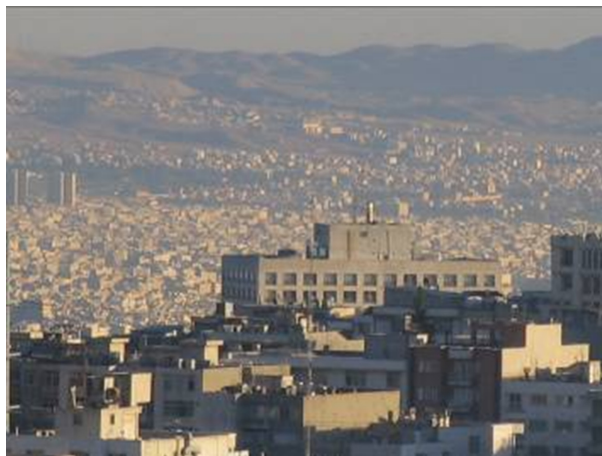
Figure 3: High density of buildings in Tehran and increasing anthropogenic heat generation.
