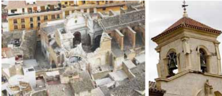
Figure 2: Historical buildings damaged in Lorca. Source: Authors.
