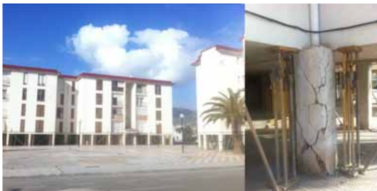
Figure 10: San Fernando district after the quake (left) and state of the columns on the ground floor (right). Source: Authors.
