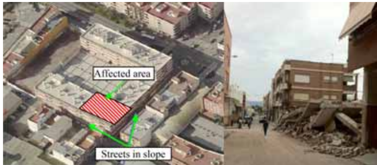
Figure 12: Location of the building collapsed in the neighbourhood of La Viña (left) and view from the beginning of the street after collapsing (right). Source: Authors.
