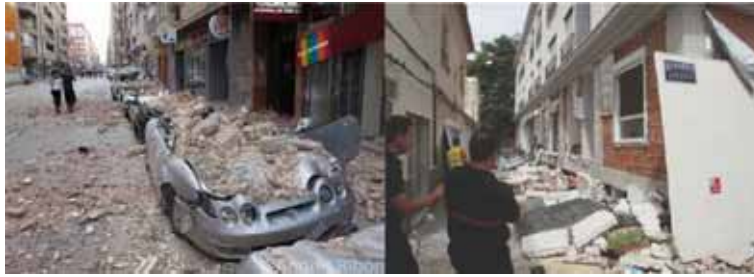
Figure 6: Detachments due to lack of bracing parapets as recommended by NCSE-02 (left) and inefficient building design (right). Source: Andrés Ribón; Authors.
