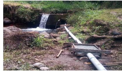
Figure 18. Penstock pipe from the fore bay reinforced with concrete slab
