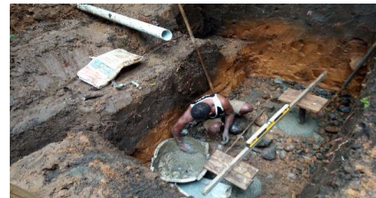
Figure 19. Powerhouse house construction
