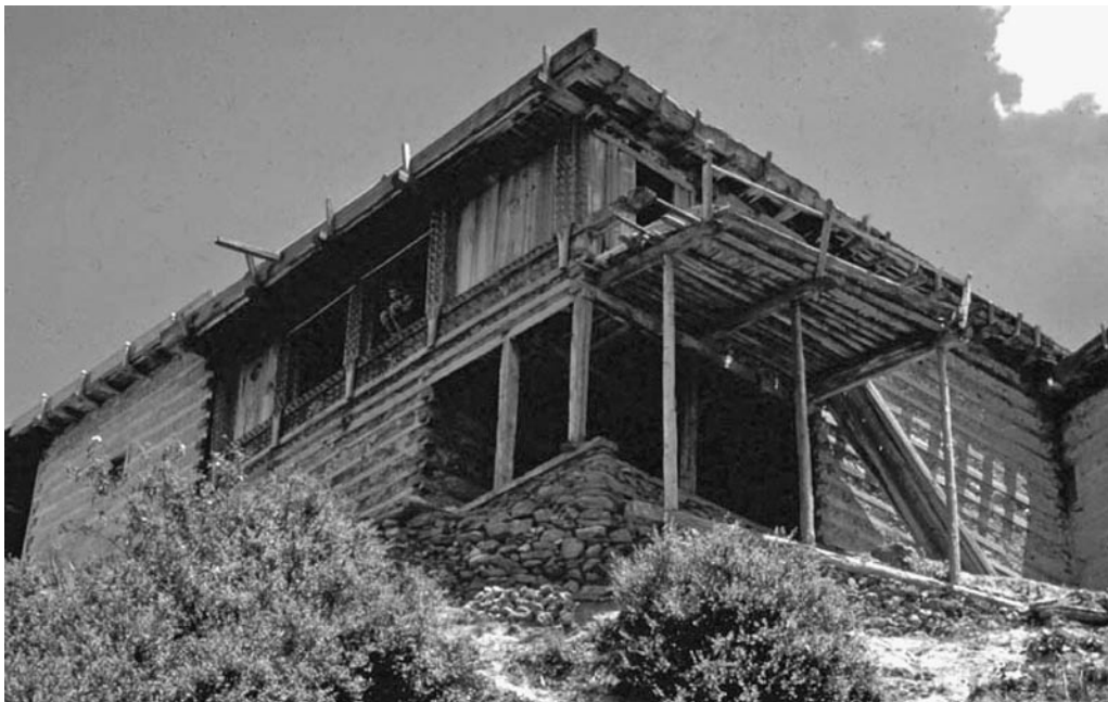
Figure 2: A two-story Nuristani house with verandah. Notice the wall construction of horizontal logs with stone fill.
