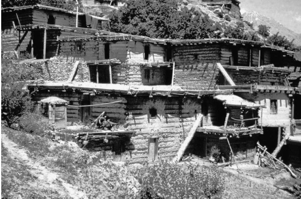
Figure 3: Typical stepping characteristic of Nuristani houses. The flat roof provides for the outdoor family space in summer. Notice the inclined log ladders that provide access to houses.
