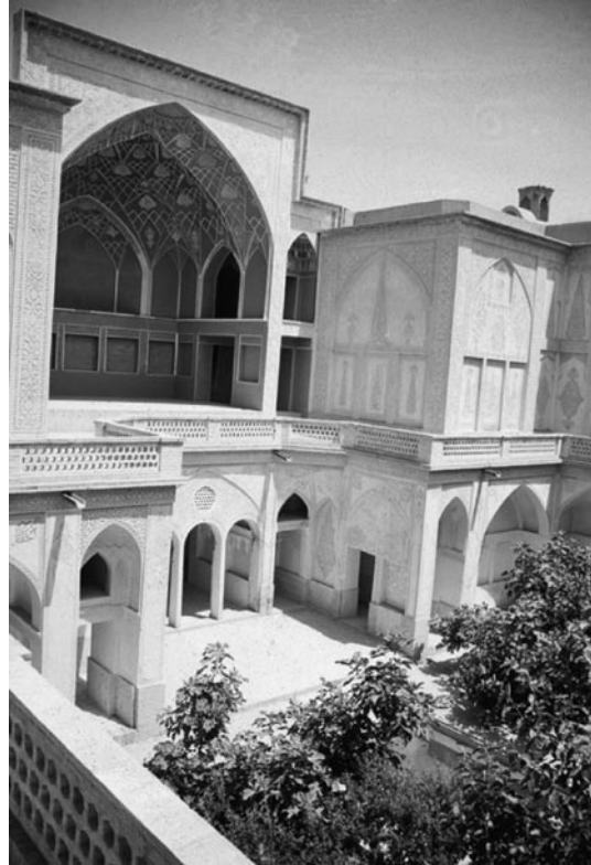
Figure 7: View of central courtyard from above. Notice the theatrical disposition of Aiwan on the upper floor.
