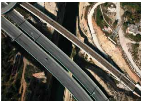
Figure 2: Elefsina (Athens)–Korinthos Motorway over Korinthos canal.
