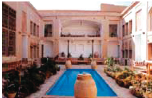
Figure 2: Courtyard with gardens and a pool in order to absorb and moderate the heat and to create a suitable microclimate inside the house.
