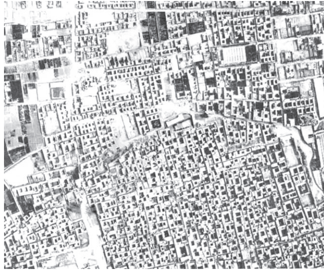
Figure 1: A city in hot-dry climate – continuous texture, attached houses, narrow streets and passage-ways (Yazd, Central Iran).
