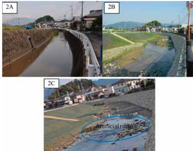
Figure 6: Station 2 condition. (A) Before restoration: a straight river lined with concrete. (B) Improvement of hydro-morphological status by re-meandering of the river and improvement of the river banks. (C) Two months after restoration; installation of artificial riffle.
