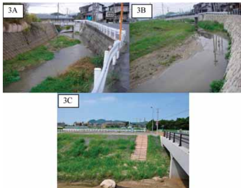
Figure 7: Station 3 condition. (A) Before restoration: concrete banks isolate the movement of organisms. (B, C) Three months after restoration: floodplain restored.
