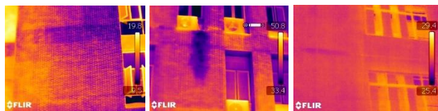
(a) Facade of Type RPPPs (b) facade of Type GHBIM (c) facade of Type RWB
