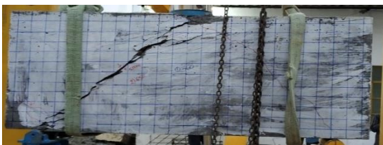
Figure 29. Ultimate loading condition 0.25%- 200 mm deep beam
