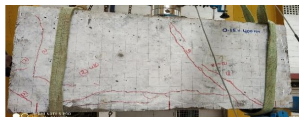
Figure 22. Ultimate loading condition 0.15%- 400 mm deep beam
