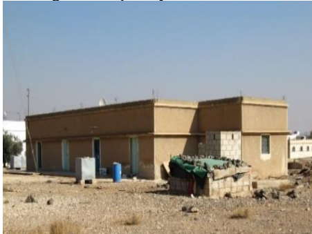
(C) Dwelling house of concrete, which represents vernacular traditional architecture
