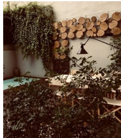
Figure 4. Green gabions at partition wall. Image from VERVEINE
