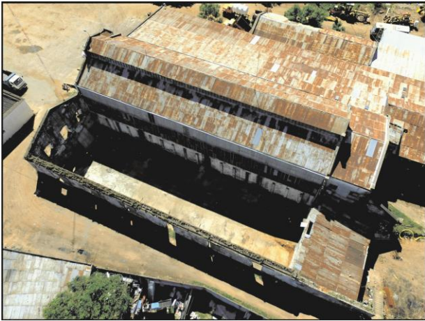
Figure 4. Harriague winery roofless shed
