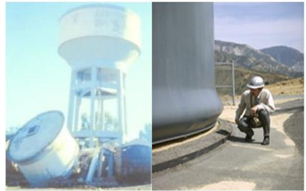
Figure 1. (a) Collapse elevated tank 1980 El-Asnam earthquake [23], Algeria; (b) Elephant foot buckling [24]
