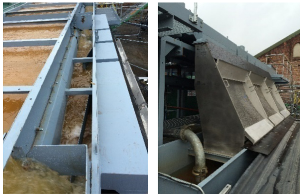
Figure 3: Structure responsible of channelling water to the plastic screens.
