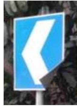
Figure 4. Damaged traffic sign
