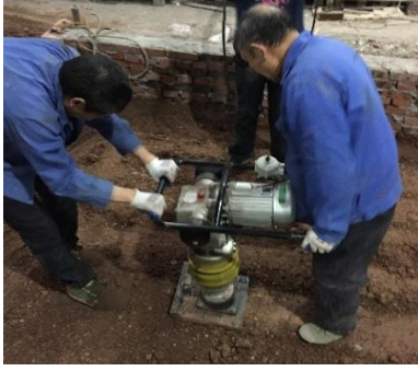
Figure 3. Layered compaction of the foundation
