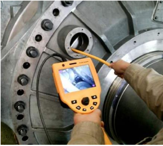
Figure 1. Internal fault detection of transformer using industrial endoscope
