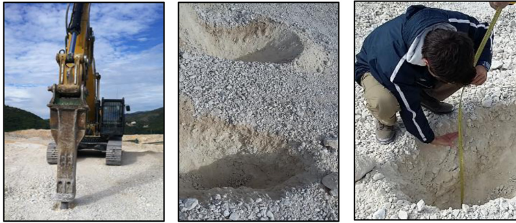
Figure 2: Excavation of the two holes for burying the transducers.
