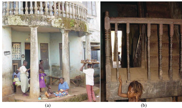
Figure 18: Ologbenla House (1), as domestic space: (a) the porch is a place of relaxation, traditional hair-dressing and interactions with trades people, among other activities; (b) a little girl at home in the staircase lobby. (S. Oluwole, 2003).
