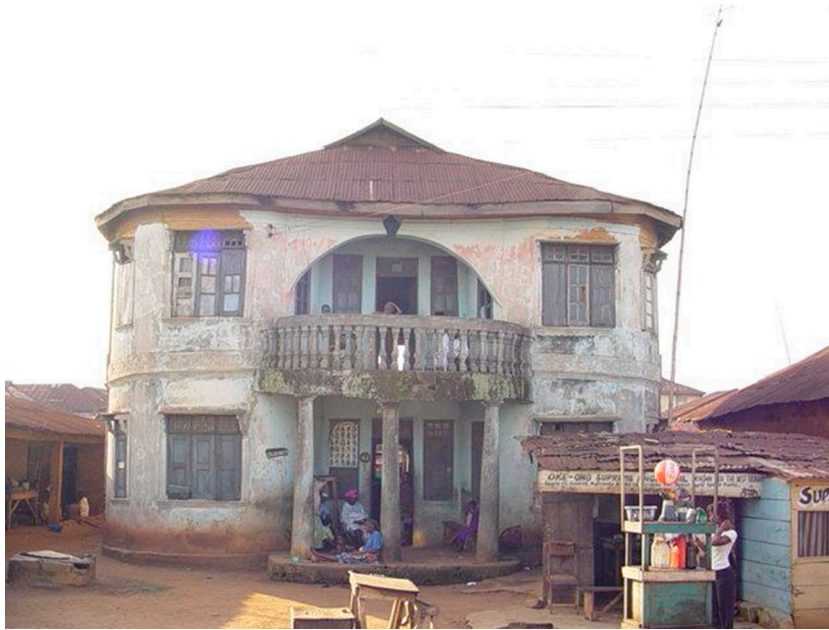
Figure 9: Ologbenla House 1. No. 55, Moore Street, Ile-Ife. View from the road. (S. Oluwole, 2003).
