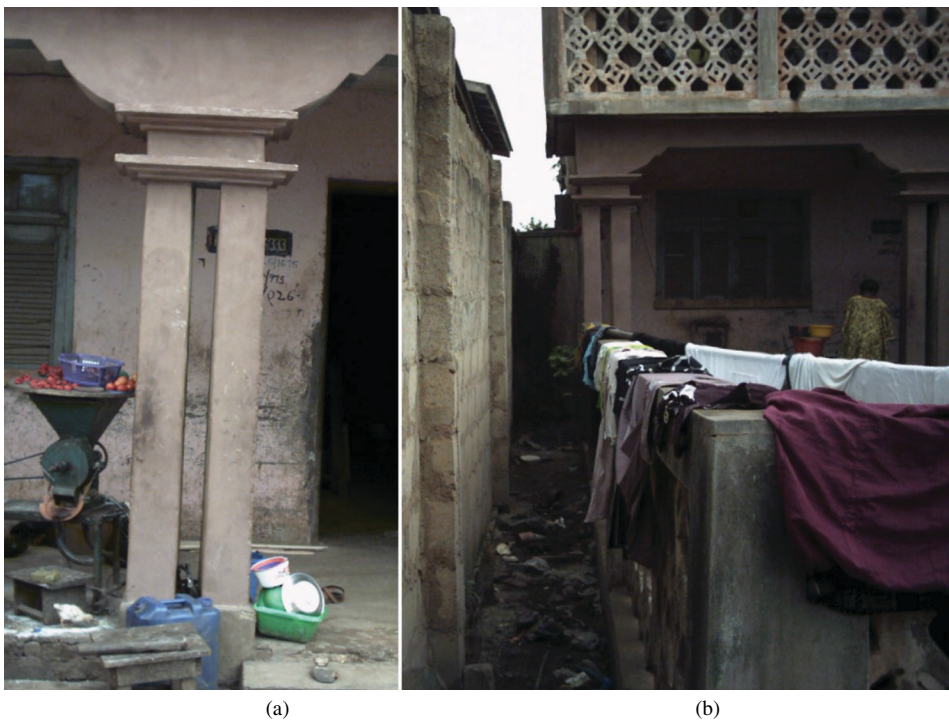
Figure 20: Evidence of domestic activity at Ile Alubarika: (a) commercial ‘pepper-milling’ on the veranda; (b) clothes spread out to dry on the perimeter fence. (A. Makinde, 2006).
