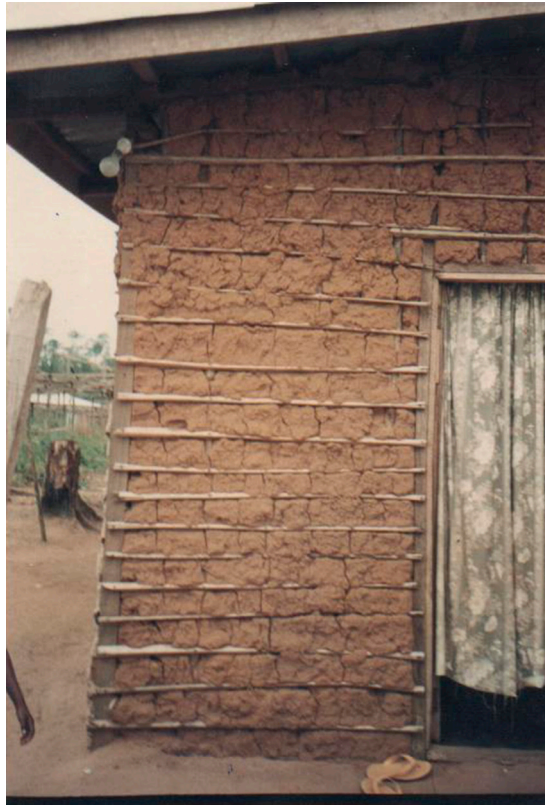
Figure 4: Wattle-and-daub construction. Eastern Nigeria. (E. Ikhuria, 2007).
