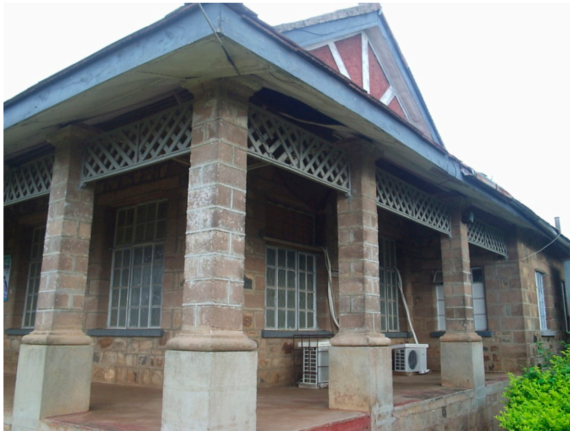
Figure 7: Saro-type bungalow, with framing veranda and timber fretwork at eaves. Modakeke, Ile-Ife. (C. O. Osasona, 2006).
