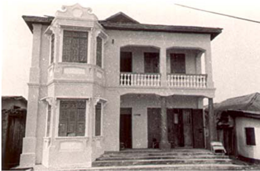
Figure 14: Ologbenla House 2, after the tentative restoration intervention in 2003. (C. O. Osasona).
