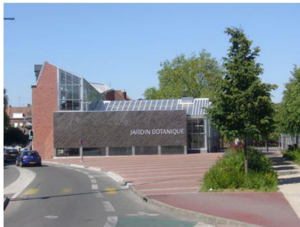
Figure 3: Greenhouses inserted in old workers houses.
