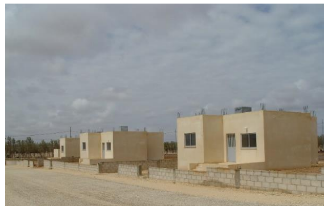
(A) Distribution of prefabricated buildings to affordable housing users
