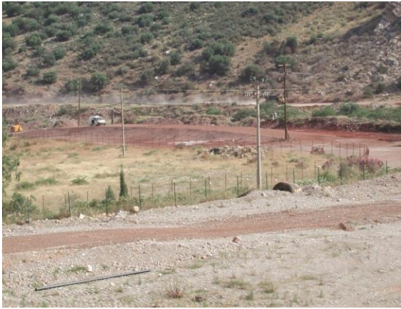
Figure 2. The experimental embankment
