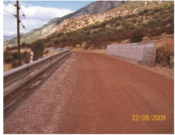
Figure 3. Initial construction of the BR road (2009)
