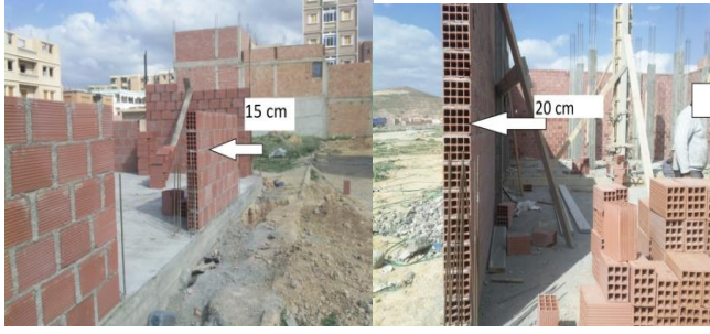
Figure 4. View of private construction
