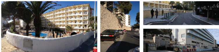
Figure 3: Street walls along the property plots in Salou.
