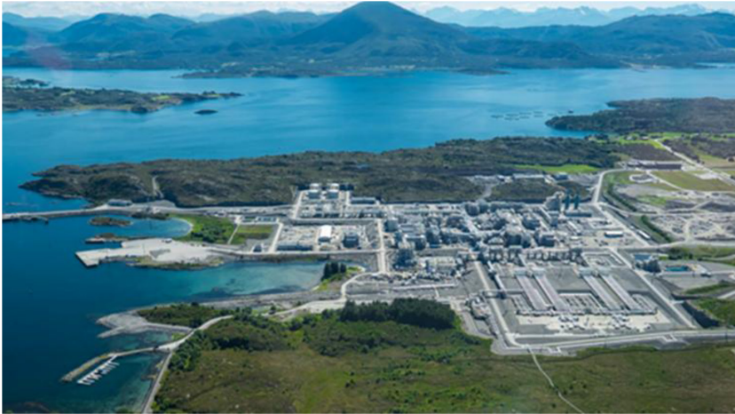
Figure 1: The Nyhamna facility
