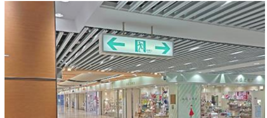
Figure 3. Conventional evacuation guide sign
