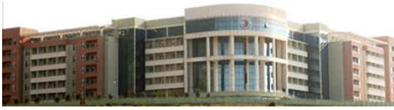
Figure 2. Image of the case building
