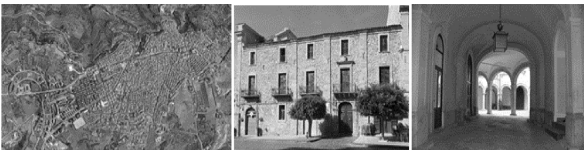
Figura 10: Mazzarino (Caltanissetta), Bartoli building, restoration work.
