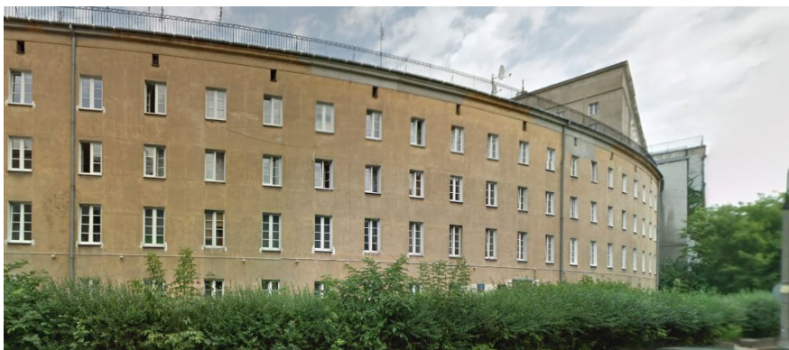
Figure 2: Muszelka Building, facade off Małachowskiego Street [authorship: Tofiluk A].
