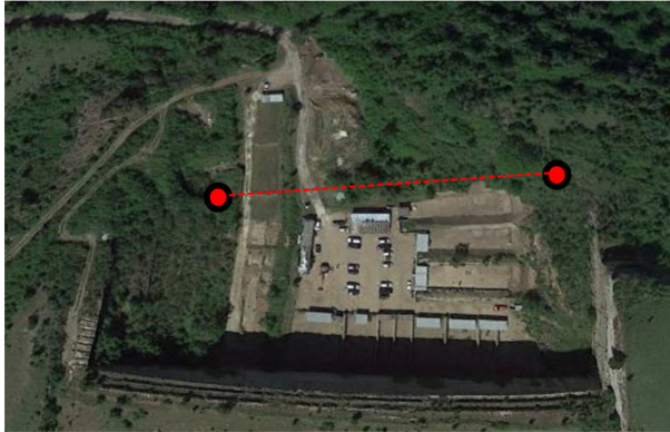
Figure 1: An aerial view of the quarry processing yard indicating the position of the high voltage cable and pylons in red.
