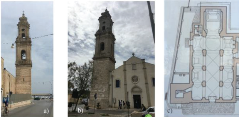
Figure 1: Bell tower of Santa Maria di Loreto (Mola, Bari, Italy). (a) North view. (b) Main façade (c) Plan view of the church with the bell tower.
