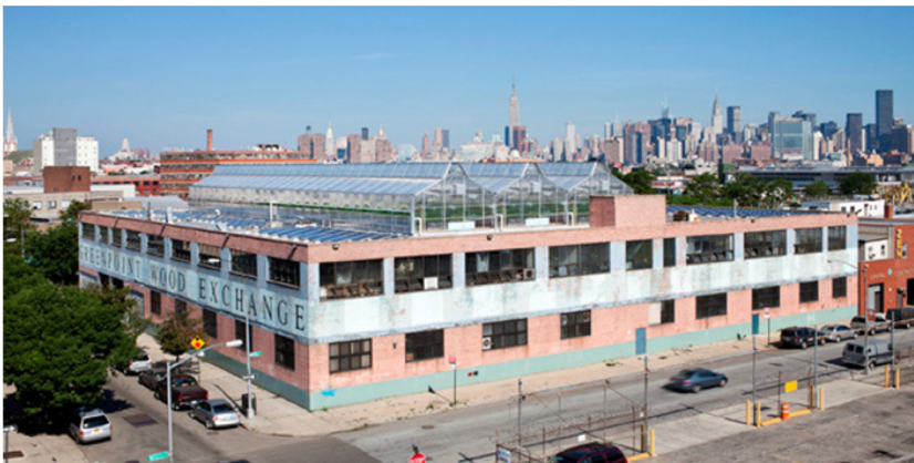
Figure 2: Greenpoint was the first commercial-scale greenhouse facility of its kind built in the United States. (Source: Gotham Greens [7]).
