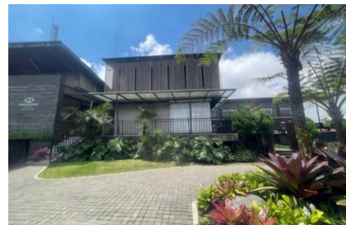
Figure 13. Timber cladding applied to the exterior façade of Pramana Zahill Kintamani, illustrating the integration of natural materials into contemporary eco-lodge architecture
