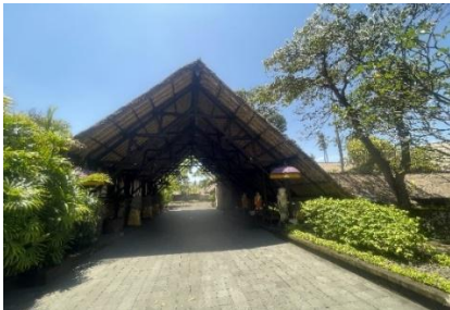
Figure 6. Traditional along-alang thatched roof and exposed timber roof structure at the main lobby of the Oberoi Resort Bali, demonstrating climate-responsive vernacular architecture
