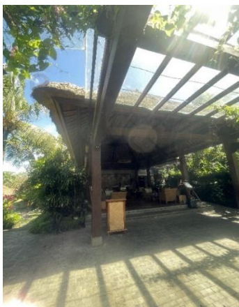
Figure 10. Alang-alang grass roofing supported by teak timber columns and timber flooring at the lobby of Adiwana Resort Jembawan, Ubud
