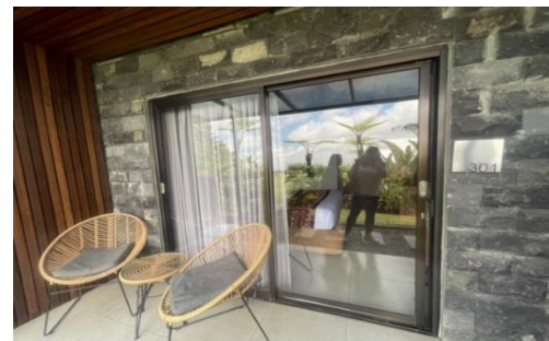
Figure 12. Volcanic-stone wall finish at Pramana Zahill Kintamani, demonstrating the application of locally available highland materials in contemporary tourism architecture
