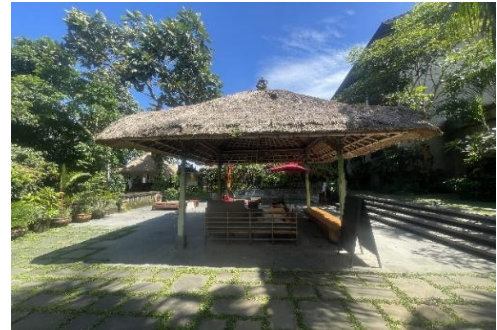
Figure 11. Alang-alang grass roofing supported by timber columns and timber flooring at the Adiwana Resort Jembawan Ubud swimming pool pavilion
