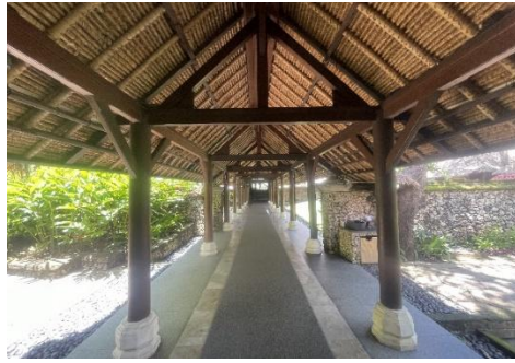
Figure 7. Exposed timber column and roof structure at the lobby of the Oberoi Resort Bali, illustrating the integration of local structural materials and traditional Balinese architectural expression
