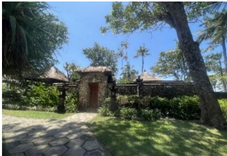
Figure 8. Jimbaran coral-stone boundary wall at the Oberoi Resort Bali, representing the application of locally sourced natural stone in Balinese resort architecture
