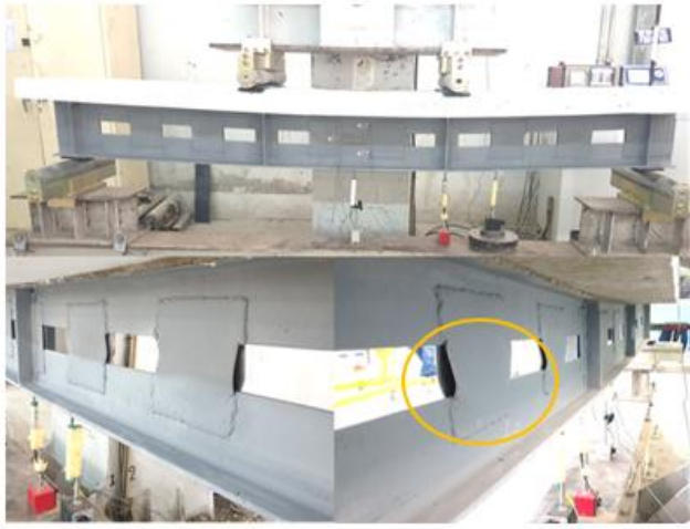
Figure 17. Failure mode of specimen B-2S.30
