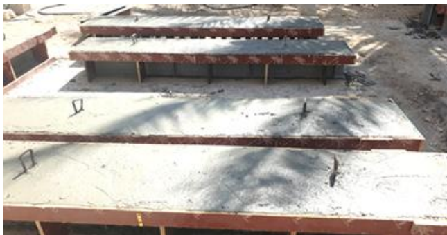
Figure 10. Casting of the test specimens
