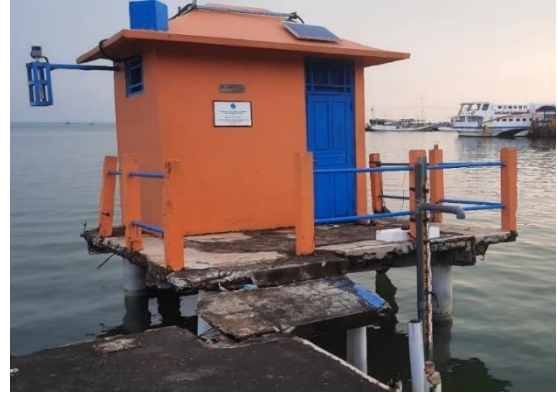
Figure 4. Installation at the test station site
