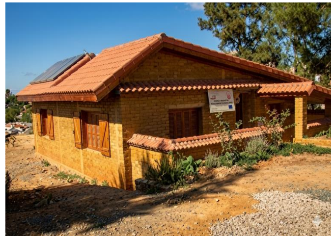
Figure 5. General view of the house (Souidania, Algiers)
