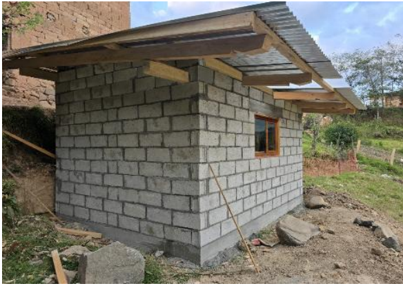
Figure 15. Construction of the module Note: 4% polystyrene beads.
