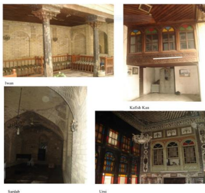
Figure 1. Main components of the traditional house in historic Al-Kadhimiya [7]
