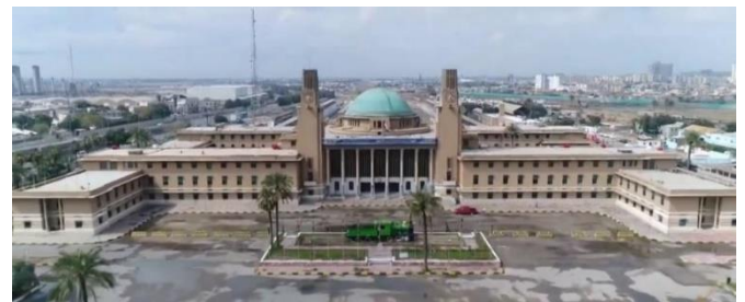
Figure 2. Baghdad Central Station [10]
