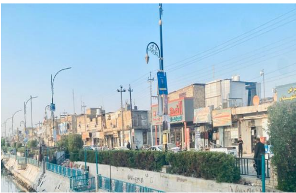
Figure 4. The river frontage on the eastern side of the Al-Gharraf River Source: The researchers
