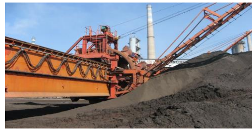
Figure 1. Wheel excavator with bridge-type bucket for the iron ore reclaiming process
