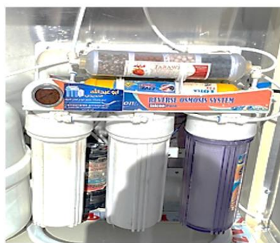
Figure 4. The main components of the brackish water reverse osmosis (BWRO) desalination
