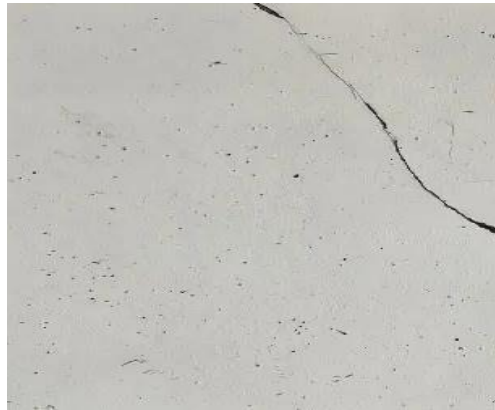
Figure 10. Tile with crack
