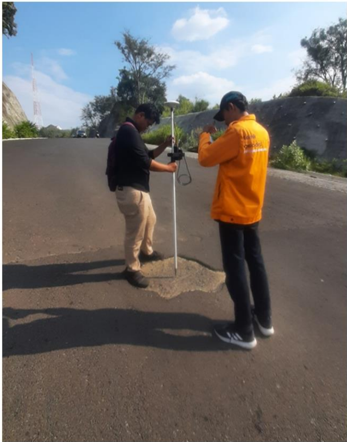
Figure 6. Implementation of verification of damage positions in the field
