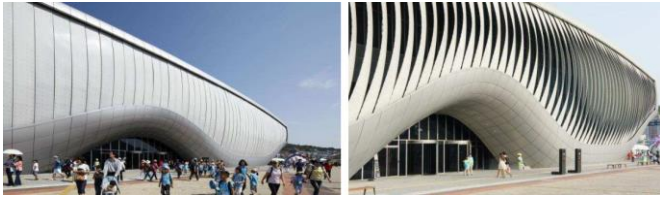
Figure 3. Closed lamellas on the left, open Lamellas on the right Architects: Soma-architecture, Vienna; Knippers Helbig, Stuttgart, New York, as the Kinetic Façade Engineer [13]
