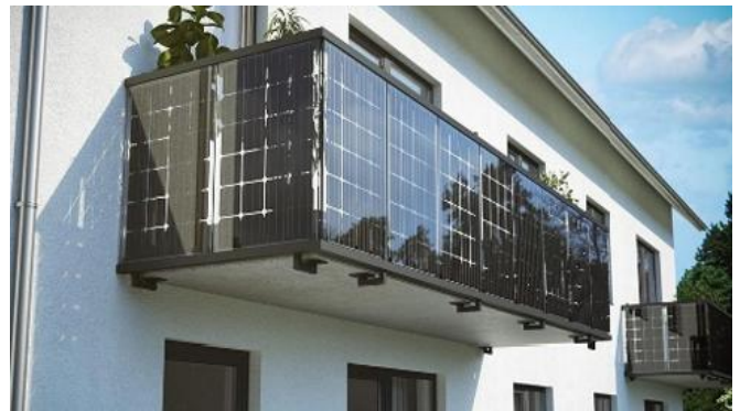
Figure 4. Applications of BIPV systems can be balconies for buildings [20]
