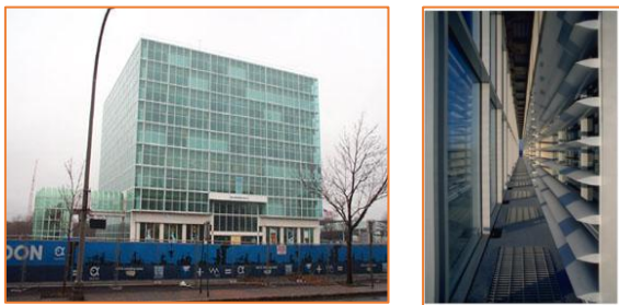
Figure 10. Solar shading louvers in the smart envelope of the Hooker Building, New York [25]
